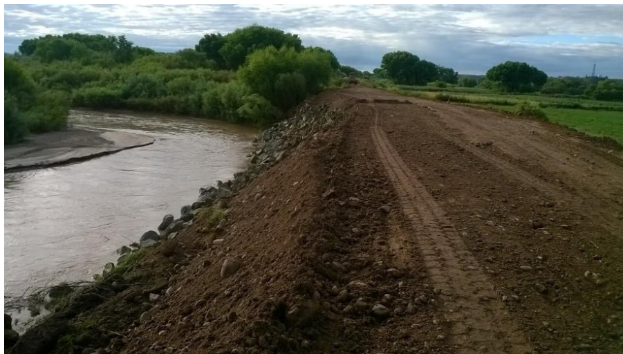
Figure 3: Current dikes in place. [16]
